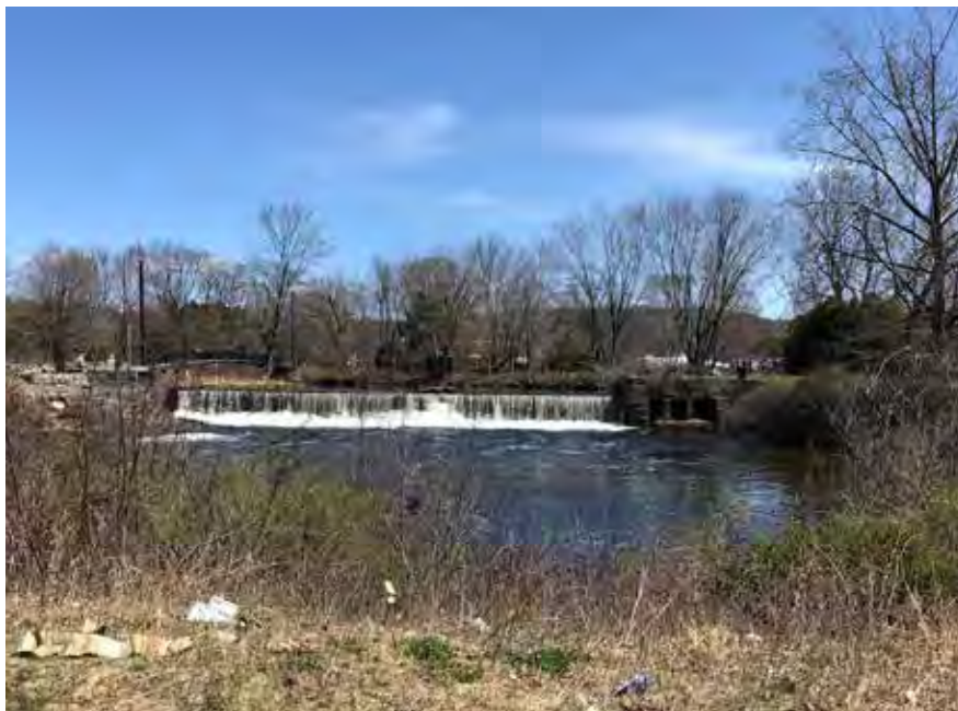
A. West Street Dam
