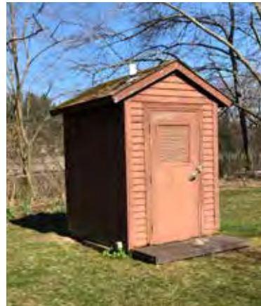
Closed composting toilet in northern Arboretum
