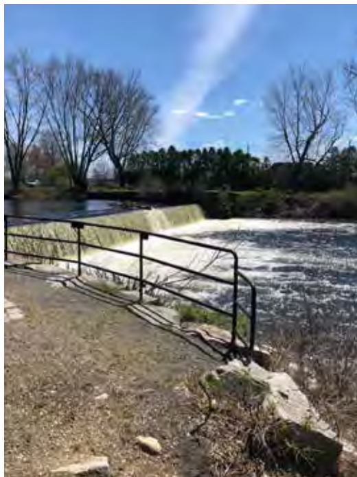
A. View of the dam
