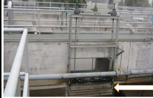
Aeration basin gate moves up and down inside the frame
