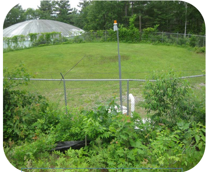
Tank is underground, inside the fence line
