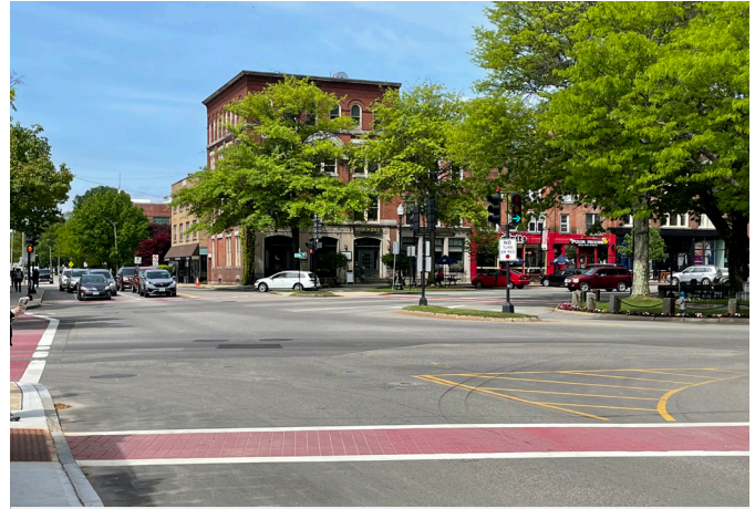
Existing street configuration near Central Square.
